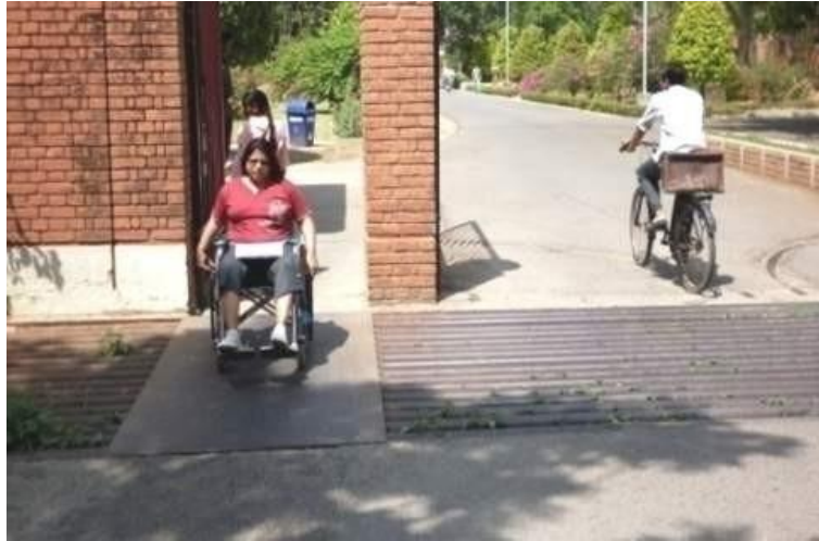
Photo 5.1 Cow catchers covered with bridge plate
