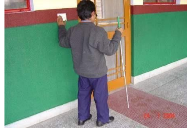
Photo 5.6 Room signage provided towards the latch side of the door
